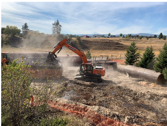
Loading scrap metal from tank #6 and #7
