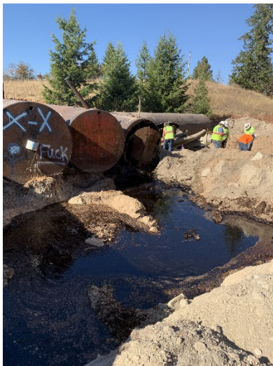
Draining of tank #7
