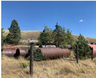
Northeast Side of Site
