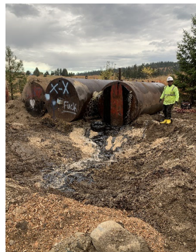
Draining of tank #8
