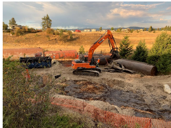
Cutting of tank #7
