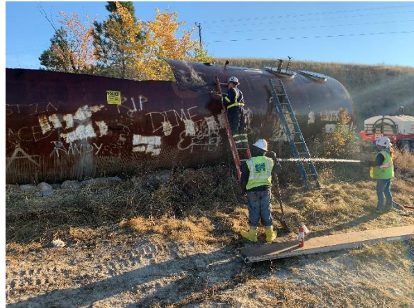
ERRS crew continue cutting tank #14
