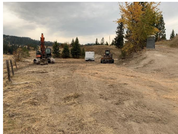
Site overview on October 21 st , post seeding
