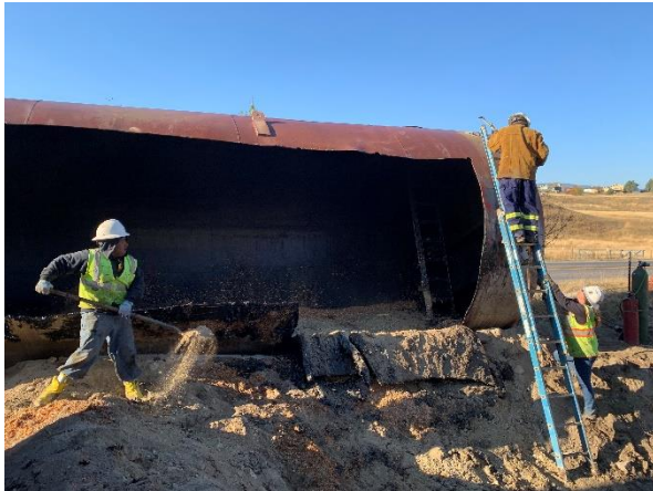
ERRS crew adds dirt for fire suppression
