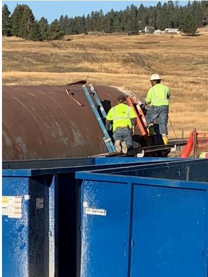
ERRS crew cutting tank #14
