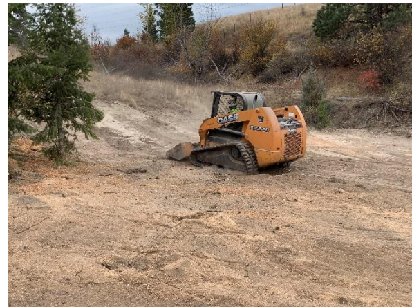
ERRS crew work on grading site
