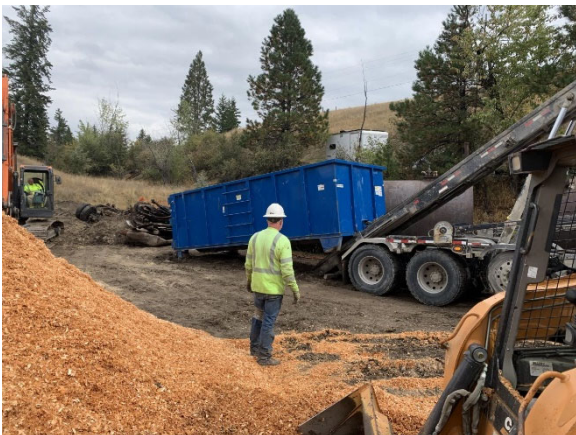
Removal of first roll-off carrying solidified waste
