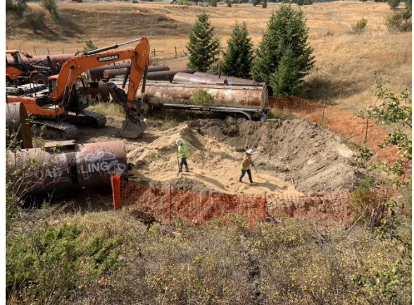
Laying of sawdust in solidification pit
