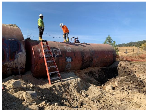
ERRS crew cutting tank #12
