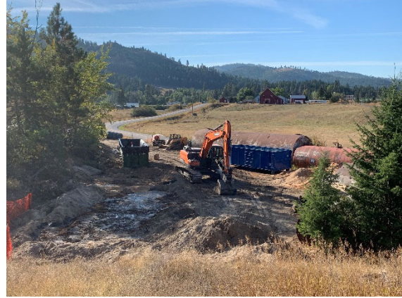
Overview of site with tanks 1-6 removed
