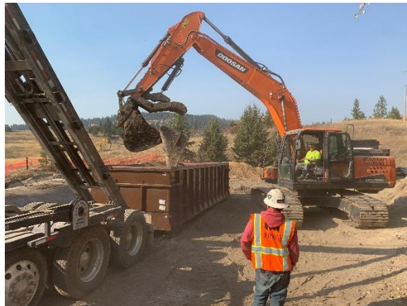
ERRS crew loading scrap metal for offsite recycling
