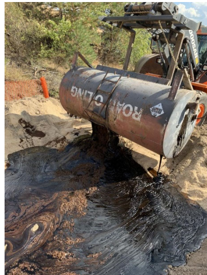
Draining of tank #2
