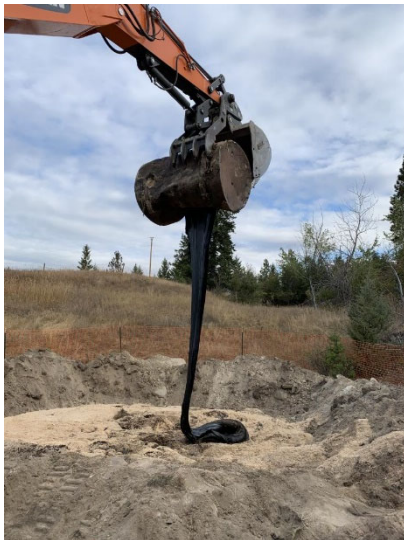
Draining of tank #1
