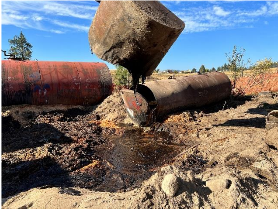
Emptying tank #9 and #10
