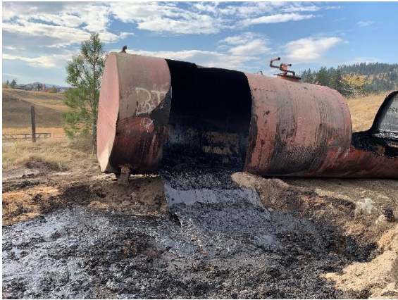
Tank #13 draining into solidification pit #2
