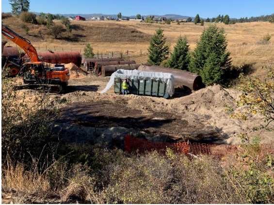
Adding poly liner to roll-off box #4
