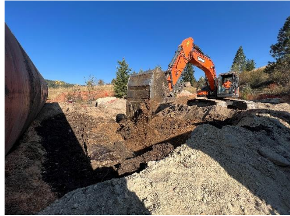
Stabilizing hydrocarbon waste with sawdust
