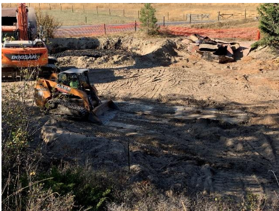
ERRS crew closing out solidification pit #1
