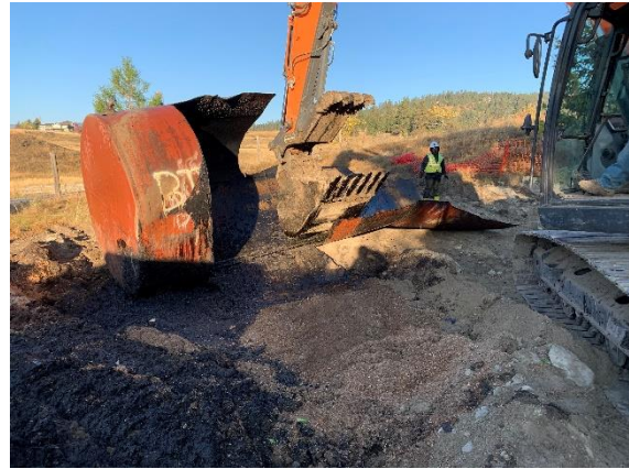
ERRS crew scraping remnants of tank #13
