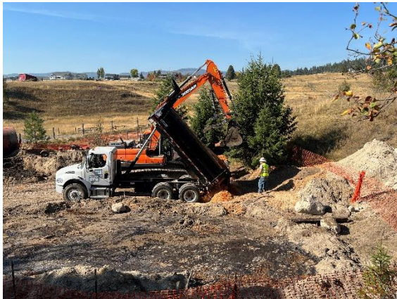
ERRS crew delivering sawdust
