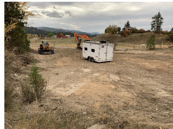
Staged equipment for demobilization
